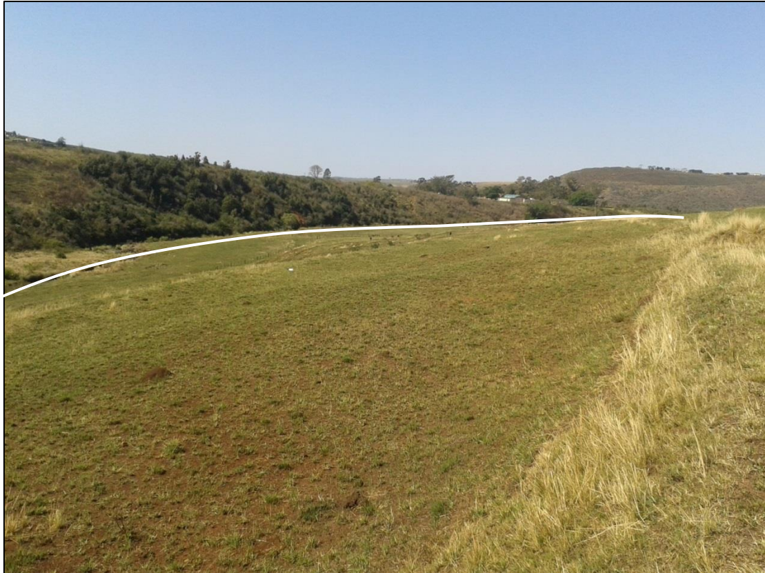
Figure 2.1: A view of a portion of the borrow pit 1 area.
